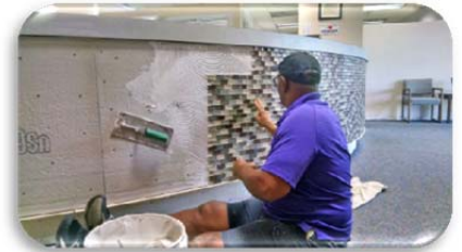
Nate Phillips installing tile in the lobby
