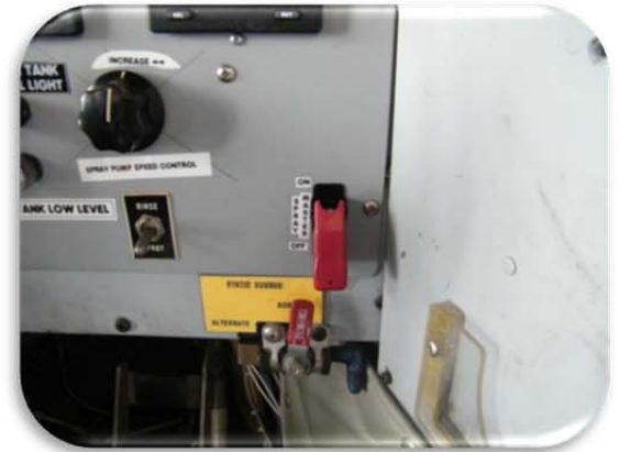
New Spray System Master Switch
